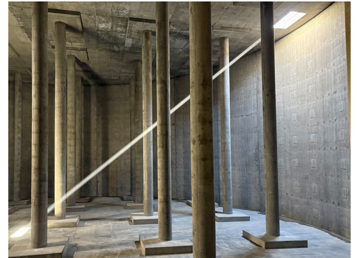
Inside of the new 4.5MG Tank.
