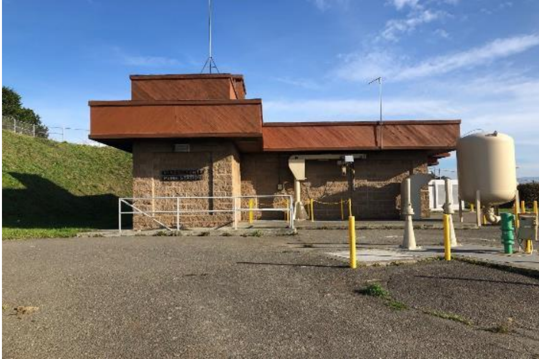
Photo 1: West Side of Fischer Station Building.
