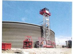
improvement in the prestressed concrete tank industry and has basically made wire wrapped systems obsolete. Because of the superiority of strand, and its predominance of use, many other advancements in prestressing technology have been coupled to the use of strand. Since there are no known patents which exist for the machine application of strand, any competent prestressing company having the necessary resources can develop strandwrapping technology.
