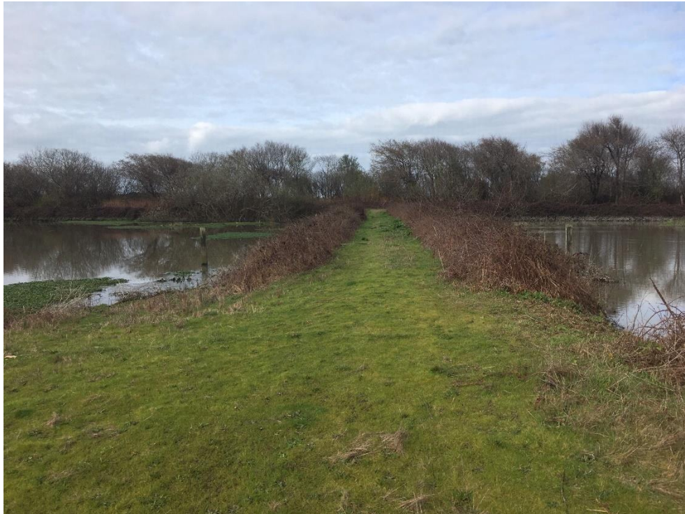
Figure 5. Existing percolation ponds shown in use in March 2018. The berm (shown) between the two ponds will be removed through project construction.
