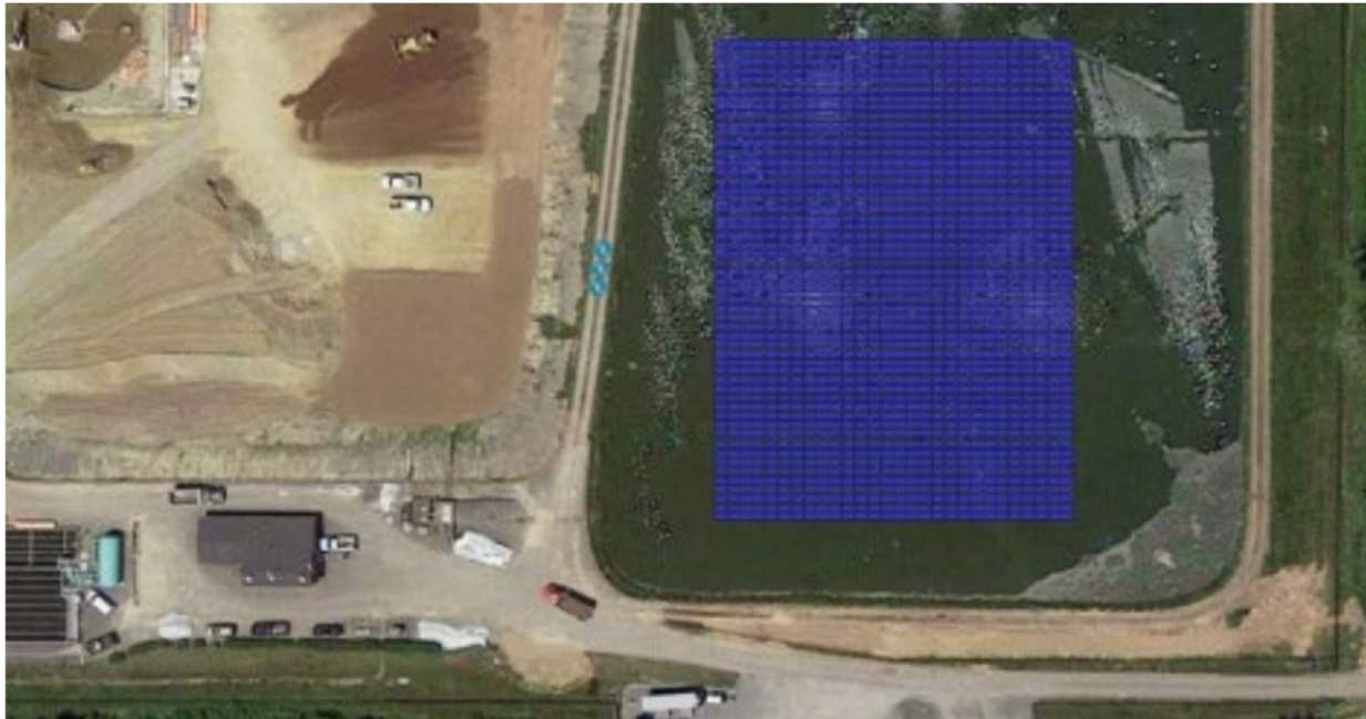
Figure 5. Floating solar array
